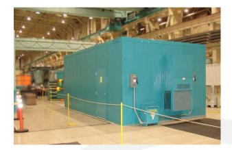
In order to properly block sound or reduce noise to predetermined levels, engineers must consider how effective the materials they choose for a barrier will be at stopping breakout noise, how spreading loss or directivity (noise loss accounted for by the direction of the noise) might determine the positioning of a barrier or where a barrier might not be needed, for example, at certain angles far away from a structure.
